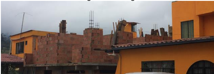
Construction of House of Retreat
